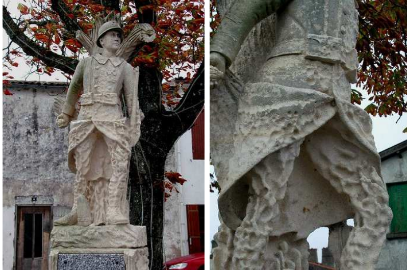
Figure 6.1: A statue of a soldier in La Rochelle (France). The legs of the statue have suffered erosion caused by salts. (Photo by Rob van Hees)
